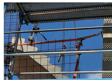
Positioning of loads
