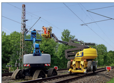
Construction of contact lines
